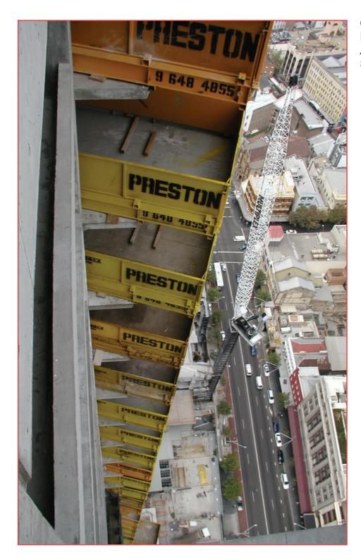
CAN BE INSTALLED DIRECTLY ABOVE ONE ANOTHER SAVING SPACE ON SITE
