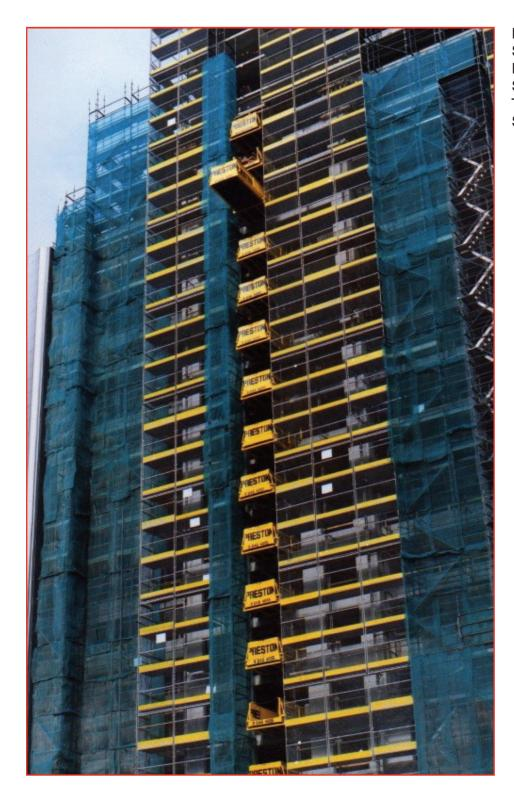
REMAINDER OF THE STRUCTURE CAN BE ENCLOSED WHILST STILL LEAVING ACCESS TO EACH FLOOR USING SUPERDECK
