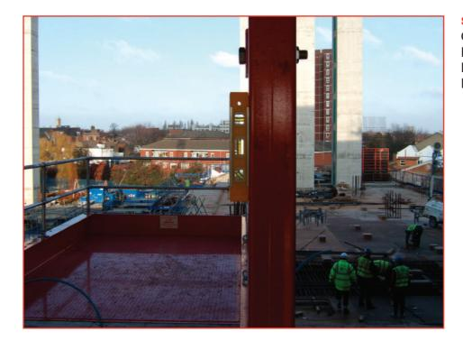
STEP 13 CHECK PROPS ARE PLUB USING A SPIRIT LEVEL AND ADJUST AS NECCESARY
