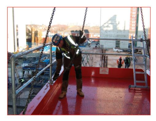
**STEP 14** LOWER OFF ON THE CRANE UNTIL THE CHAINS COME LOOSE
